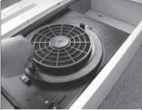
1. Pull up and twist the two spring loaded clips around the carbon filter holder.
