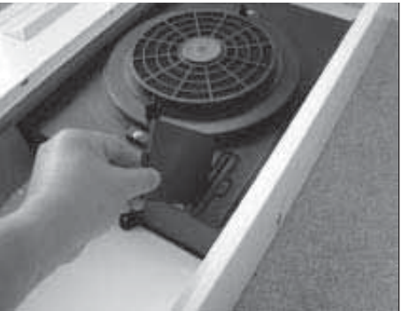
3. Insert air diverter plate and screw into place.
